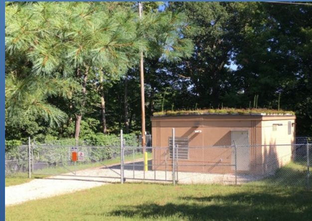
Greenland Well Replacement and New Pumphouse 2018 648,000 Gallons-per-Day
