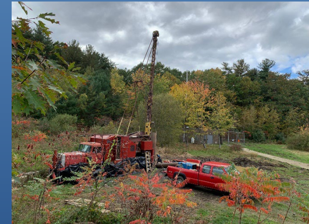
Collins Well 2 2021 (ongoing)
