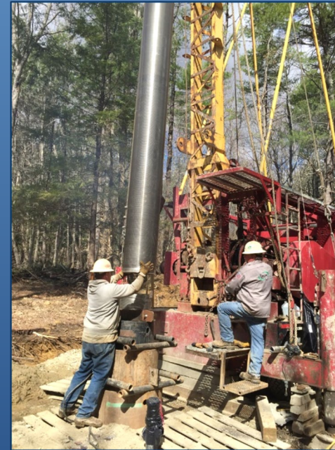
Madbury Well 5 Installation and Permitting 2018 720,000 Gallons-per-Day
