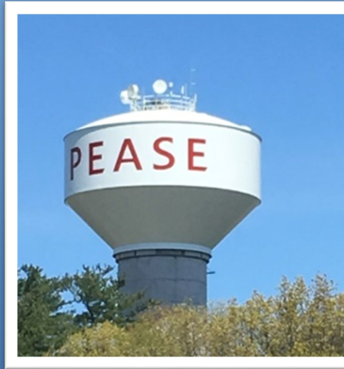
Pease Water Tank - 2016
