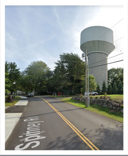
Spinney Water Tank - 2002
