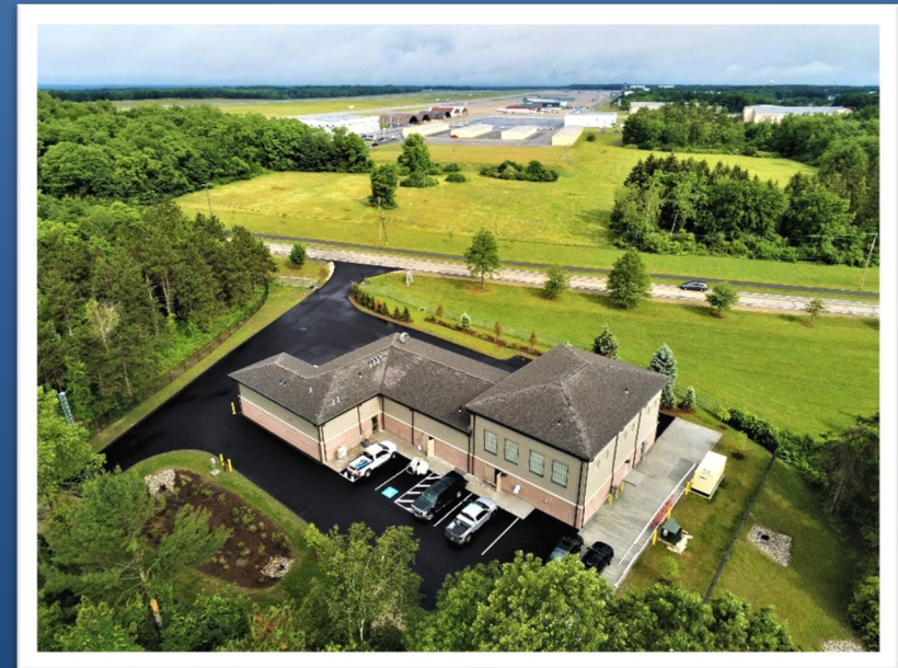
Pease Water Treatment Facility - 2021
