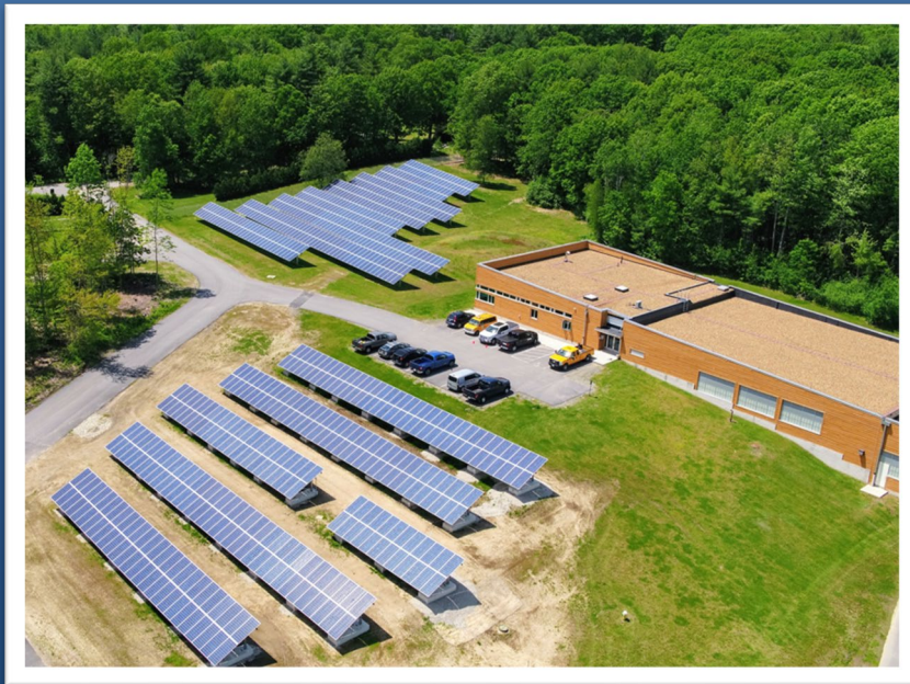
Madbury Water Treatment Facility - 2011
