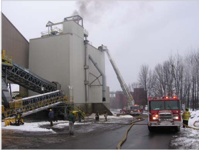
PSNH Wood Processing Plant fire on February 28, 2011
