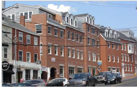
The Martingale Wharf project on Bow Street
