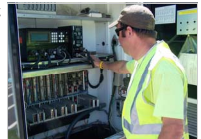
Checking traffic control equipment
