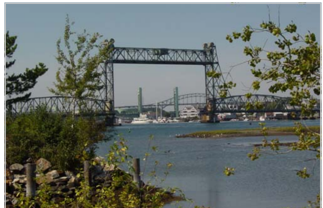
The replacement of the Memorial Bridge between Portsmouth and Kittery, Maine, is important to local and interstate commerce
