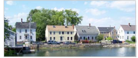
South Mill Street seawall reconstruction
